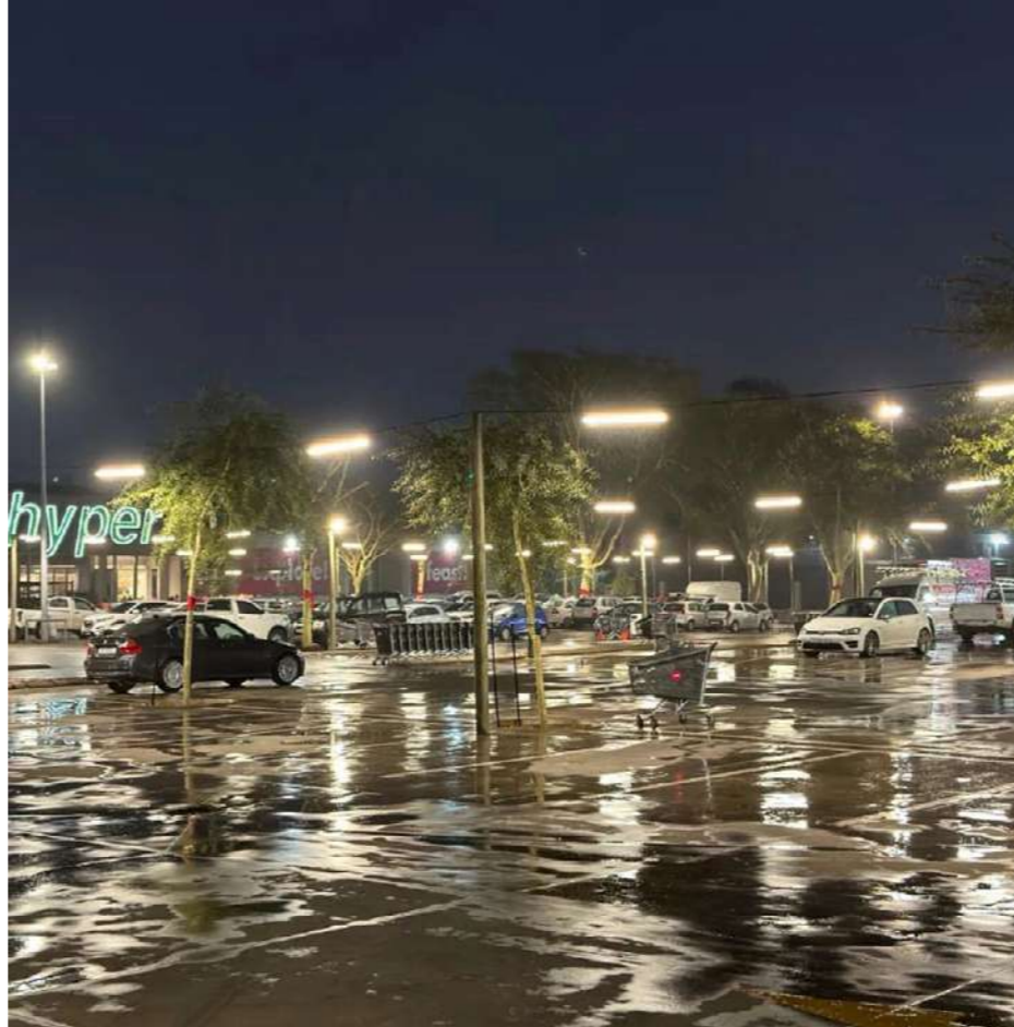
Something different from EuroConcept's normal brief ... suspended luminaires were used as a car park lighting solution at Save Hyper in Pietermaritzburg. https://euroconcepts.co.za/
