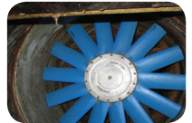
Sample - Kitchen Extraction System
